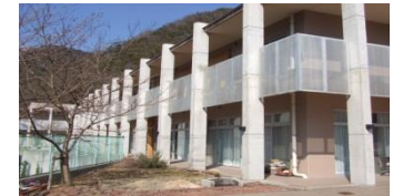
Fukayaso, Nursing Home in Okayama
