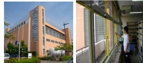
Tokyo Gakkan Niigata high school
