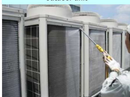
High pressure washing for the outdoor unit
