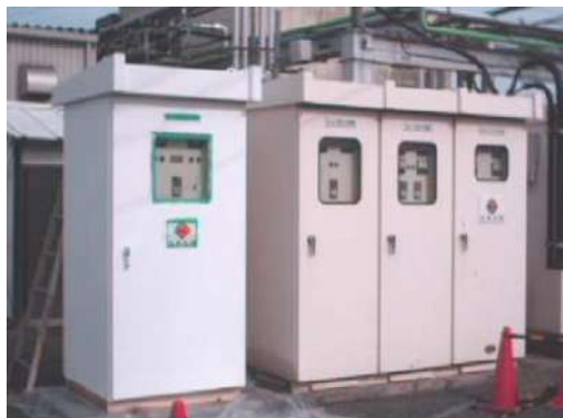
③ cubicle type high voltage receiving equipment
