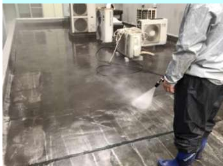
High pressure washing on the roof
