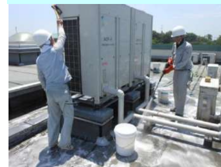
Oil washing on the Floor surface
